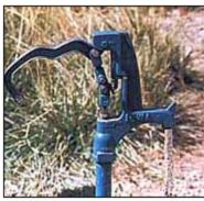
To turn the water on, you simply raise the lever up to the ON position. As long as the lever remains in the ON position, the water flows continuously. The photo at left shows the lever in the up or ON position.
